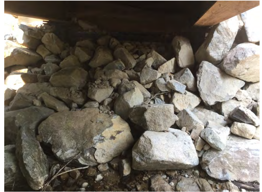
Right Bank Abutment when facing downstream
