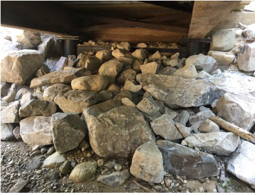
Left Bank Abutment when facing downstream
